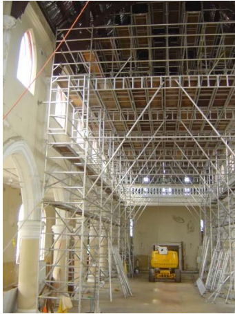
Mother of Good Council Church, Innisfail, Scaffold certification.
