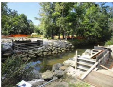
Warrina Lakes bridge re-construction
