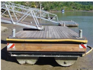
Russell River Pontoons, regulation compliance inspection
