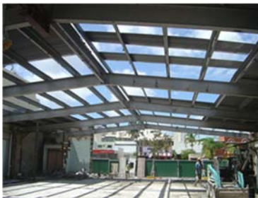
Portal frame de-construction and re-location
