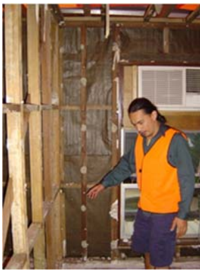
On an inspection
