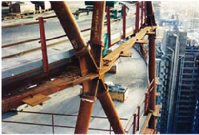
Iconic Swiss Re building under construction (the Gherkin) City of London.
