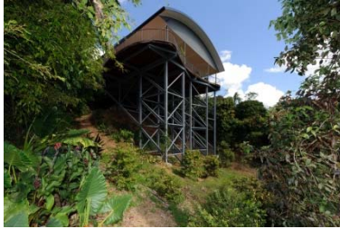
Teece Residence, Earlvile, 26m propped span over steep slope. 2011 HIA Australian Finalist
