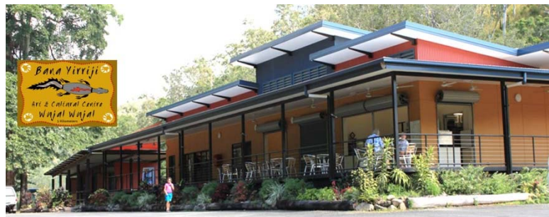
Bana Yirriji Arts and Cultural Centre for the Wujal Wujal Aboriginal Shire Council 2014 Regional BDAQ Award winner: Public Building. Finalist Australian Building Design Awards.
