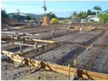
Social housing Thursday Island, construction inspection and certification.
