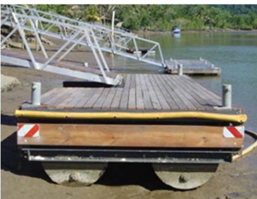
Russell River pontoons, regulation compliance inspection
