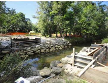
Warrina Lakes bridge re-construction
