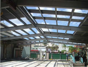
Portal frame de-construction and re-location
