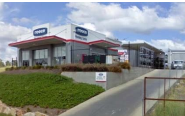
Reece Plumbing Centre, Jimboomba
