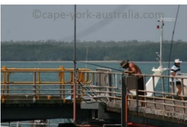
Evans Landing, wharf extension, Weipa
