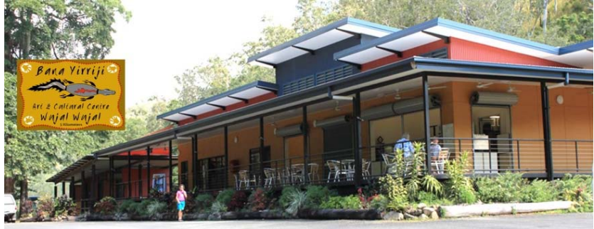
Bana Yirriji Arts and Cultural Centre for the Wujal Wujal Aboriginal Shire Council 2014 Regional BDAQ Award winner: Public Building. Finalist Australian Building Design Awards.
