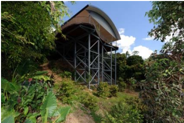
Teece Residence, Earlville, 26m propped span over steep slope. 2011 HIA Australian Finalist
